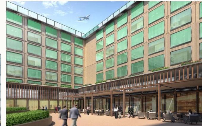
Prestige Trade Centre (Under Construction)
