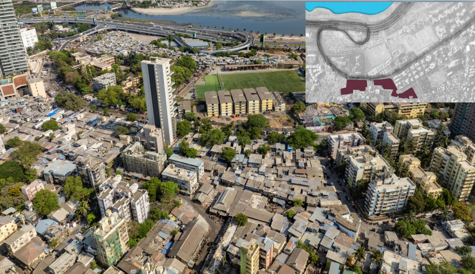
Project Area - Aerial view
